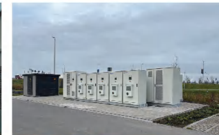
Garden Center, Netherlands Capacity: 1MW / 2.2MWh Application: Solar Self-consumption
